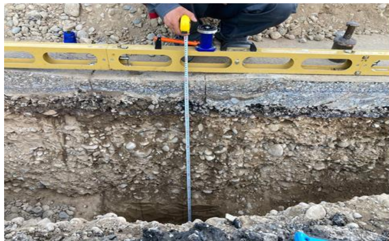
FIGURE 2. Measuring thicknesses of the pavement layers
