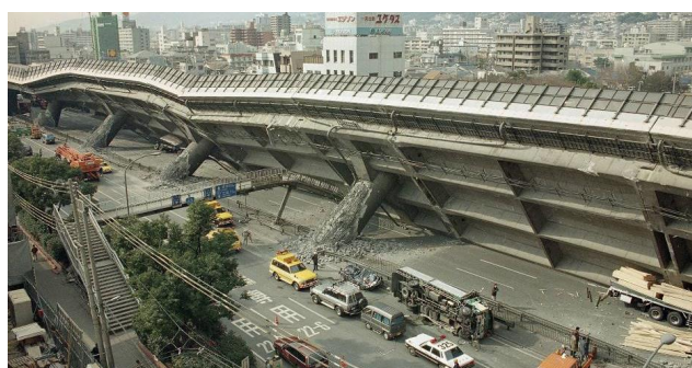
FIGURE 2. Higashi-Nada Viaduct collapse in the 1995 Hyogo-Ken Nanbu earthquake. (Source: EERI, The HyogoRen Nambu Earthquake, January 17, 1995, Preliminary Reconnaissance Report, Feb. 1995.) [4-7]
