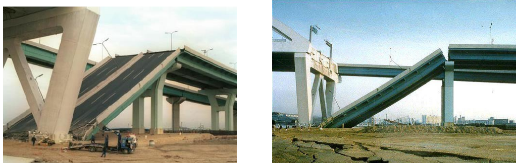
FIGURE 1. Nishinomiya-ko Bridge approach span collapse in the 1995 Hyogo-Ken Nanbu earthquake (Kobe Collection, EERC Library, University of California, Berkeley) [4-7]
