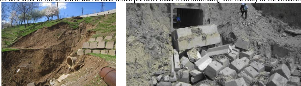
FIGURE 2. Road sections damaged due to loss of foundation bearing capacity, Uzbekistan (Photo by Abirov R.)
