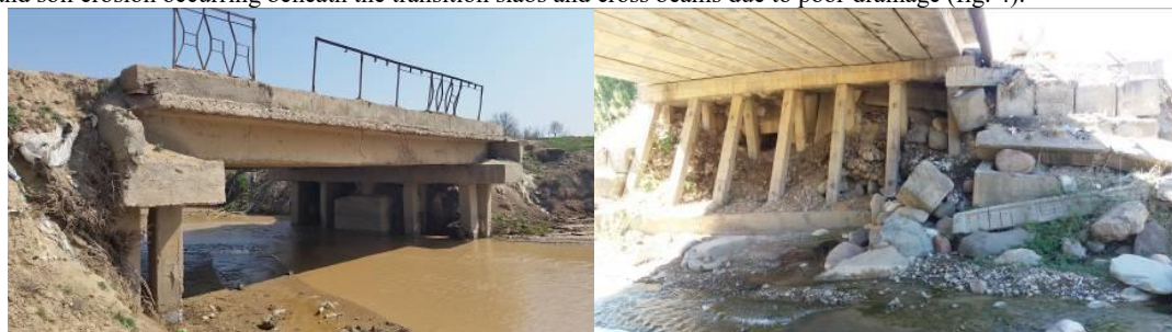
FIGURE 4. Soil subsidence due to insufficient compaction and soil washout from under transition slabs (Photo by Abirov R.)
