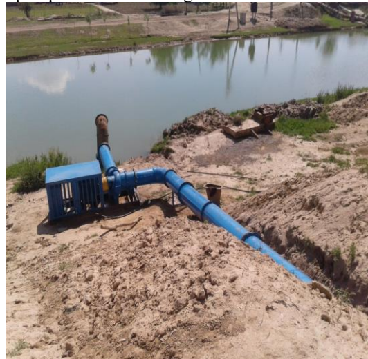
FIGURE 2. Full-scale testing of D3200-75 pumps; a) characteristics of the D3200-75 pump; b) location of the pumping unit.
